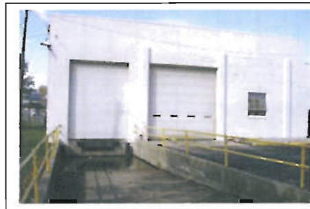
East Receiving Area
